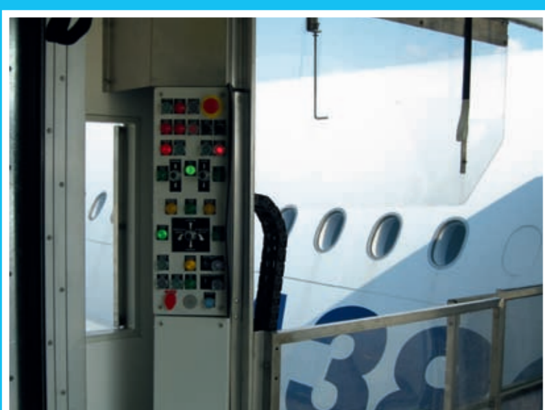
Control panel on the platform
